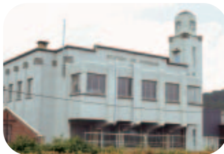
Station de pompage.
